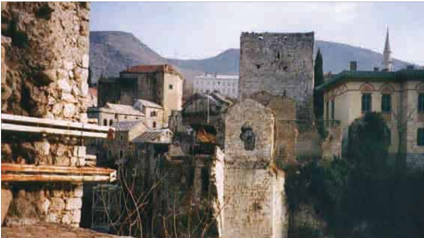
The bombed and destroyed bridge at Mostar, Bosnia and Herzegovina, 1993. Photo: Jon Roar Strandenes
